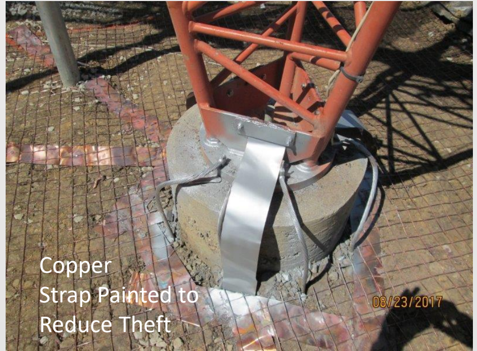
Only 2.43 amps vs. 60 amps RF previously
