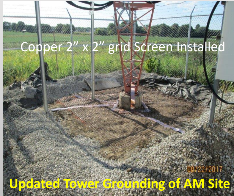
Copper Strap was Extended to Building
